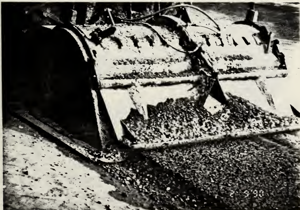
Figure 2.18 Wet Mixing of Aggregate and Cement Powder
